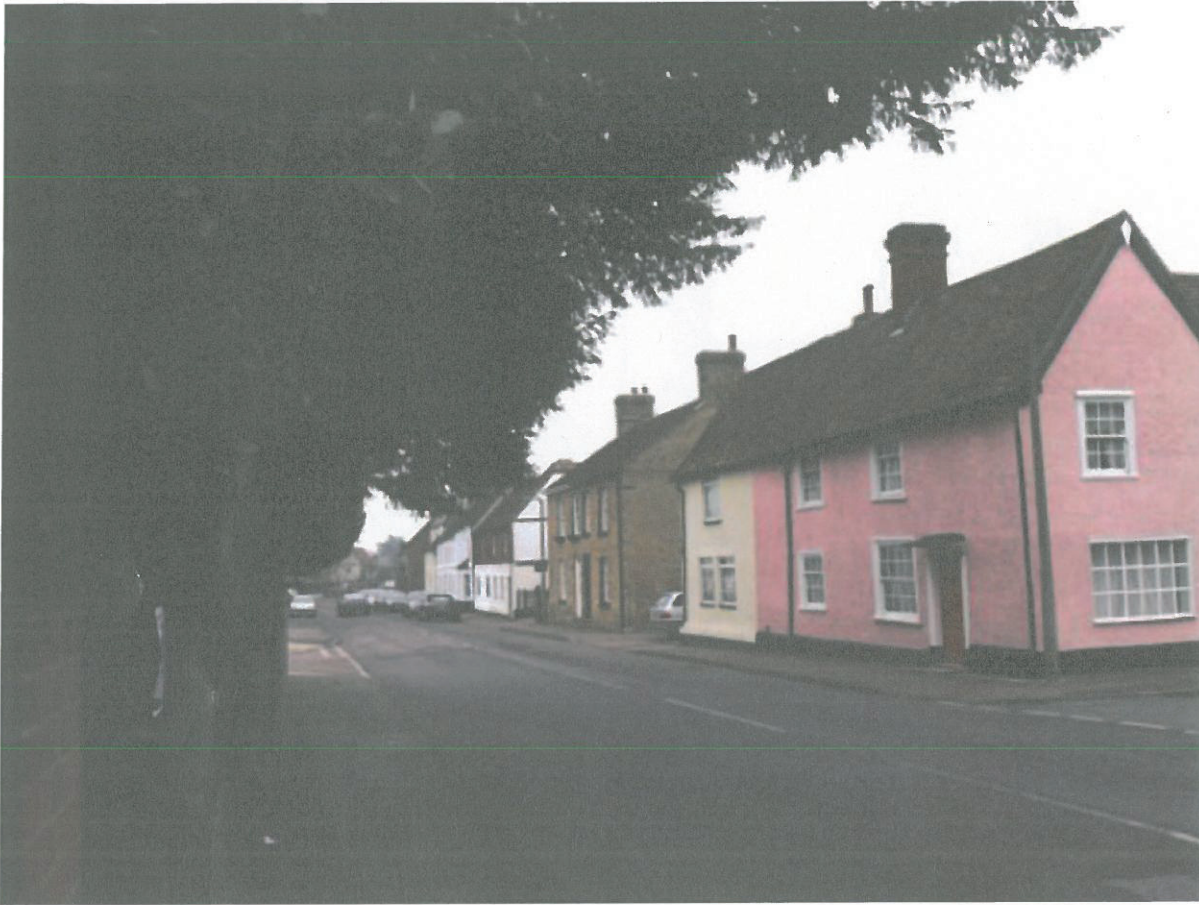
Figure 3: Maypole House (Grade 2 Listed).
